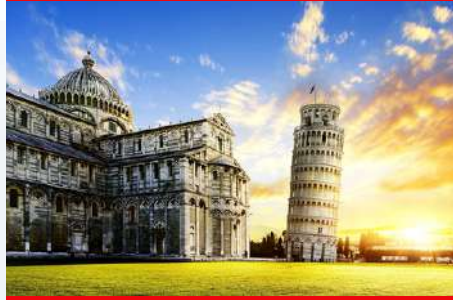
Leaning Tower of Pisa
