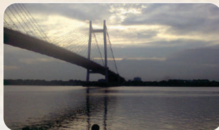
Vidyasagar Setu is the first and longest cable-stayed bridge in India and one of the longest in Asia.
