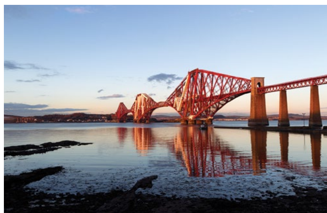
Firth of Forth Rail Bridge
